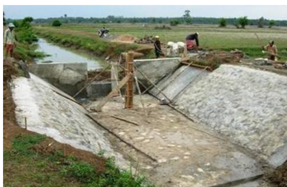
Figure 19: Check-structure in Pram Kumpheak
