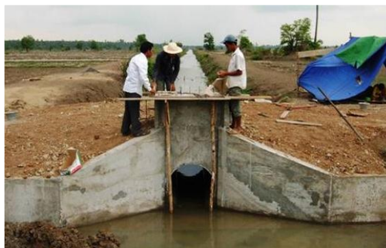
Figure 18: Culvert (II canal), Pram Kumpheak scheme
