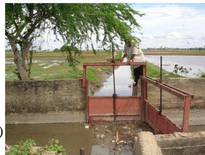
Sluices (N°4 and 5) on primary Canal
